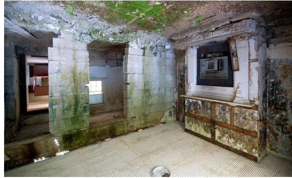
Plate 55: Inside Cottage prior to renovation (Source: Wollondilly Council).
