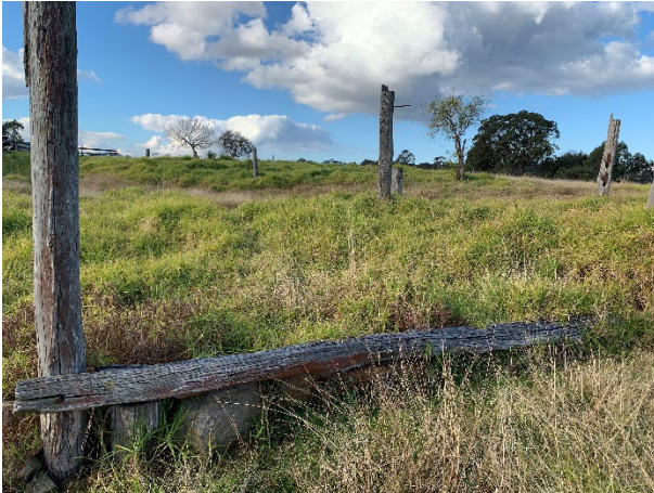
Plate 33: Timber poles and cross beams, overlying rough sandstone footings. Facing north-east.
