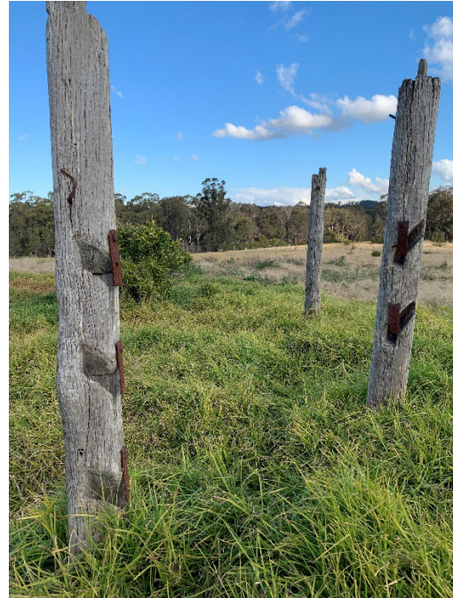
Plate 34: Poles with mortice joints. Facing south-east.
